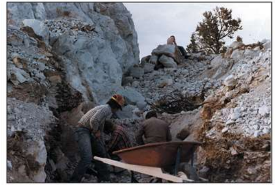
Figure 2. Early work consisted of blasting, pick, shovel and wheelbarrow work.
